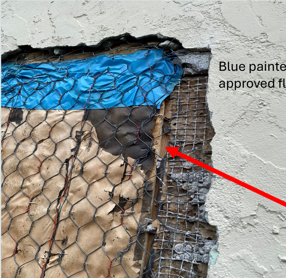
CRC R703.7: Exposed plywood and framing seen during pre-stucco inspection
